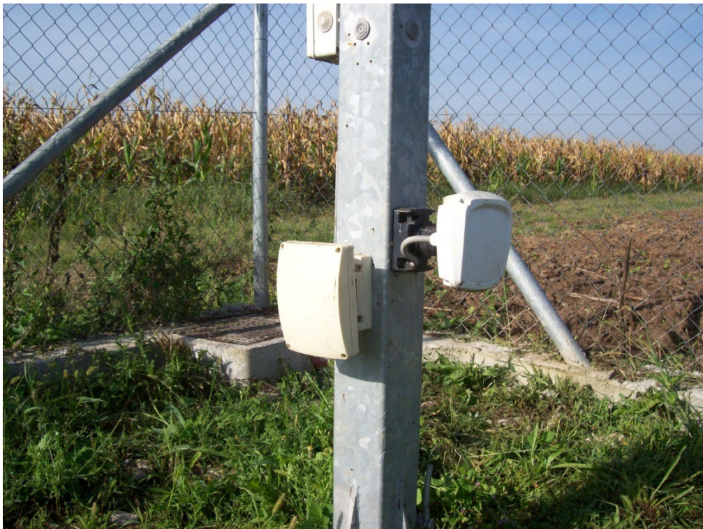
Right: Microwave Detector 150m, Left: Microwave Detector 220m.
